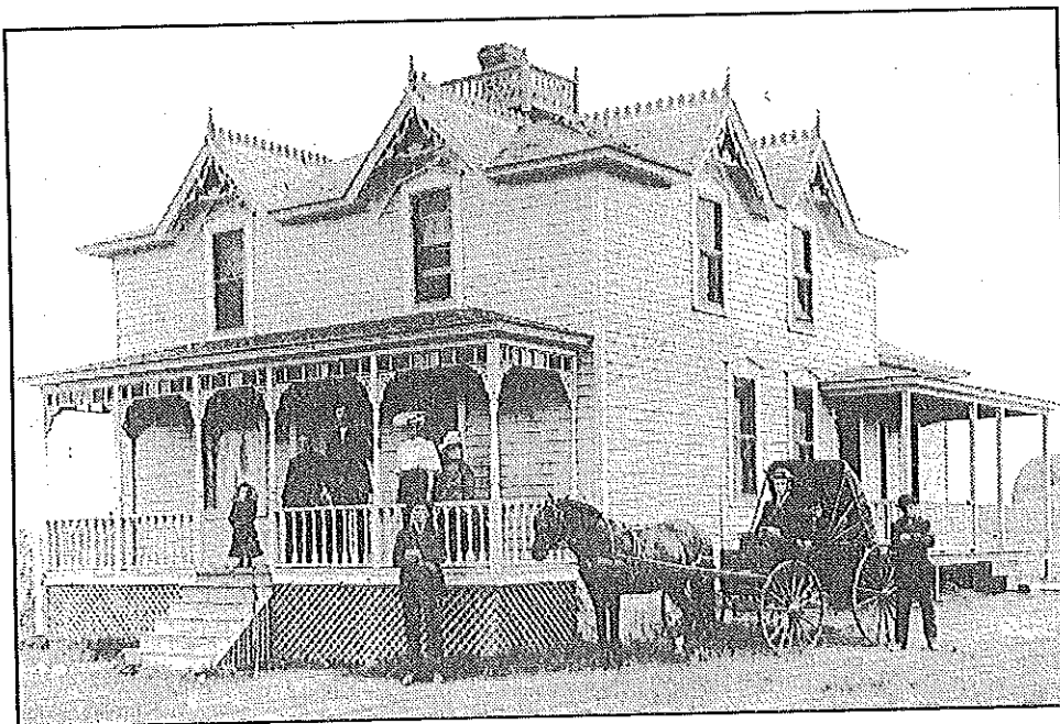
Courtesy photo Shown is the original Bentz house, built by Jakob Bentz in 1905. The house is still standing.
